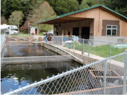
Photo 3: Morgan Creek hatchery building under construction
