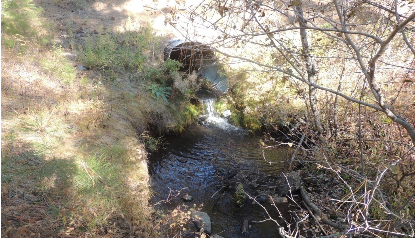
Photo 8 Union Creek Culvert
