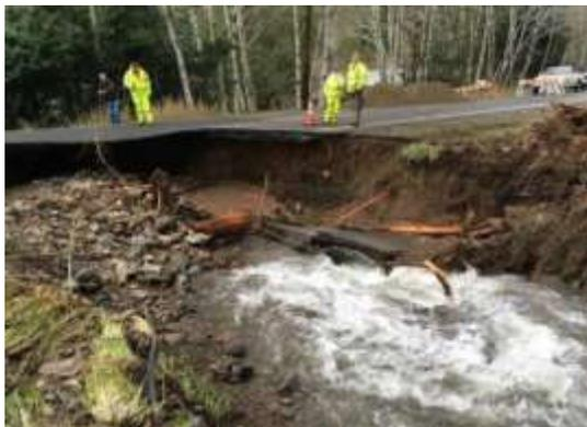
Culvert washout on Miami Foley Road in north Tillamook County. No road fill was left under the suspended asphalt.
