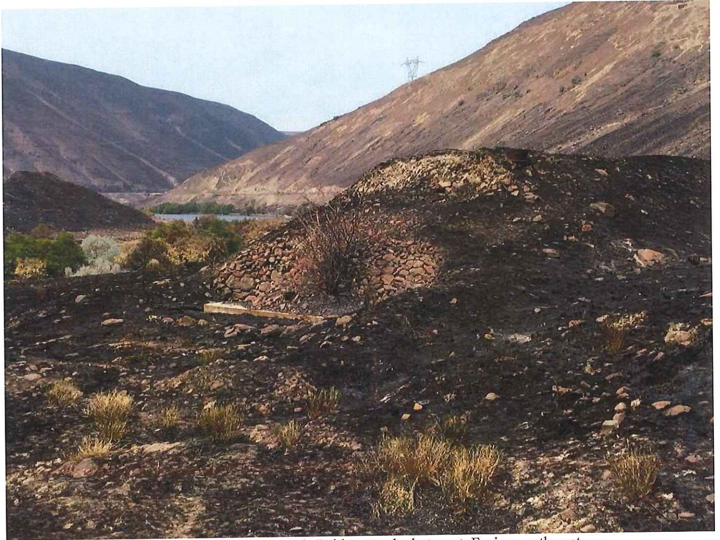
Figure 6. Rattlesnake Grade Bridge, north abutment. Facing northwest.
