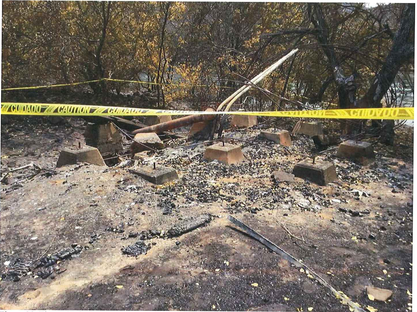
Figure 20. Figure 19. "River Mile 12: Deschutes River Harris Ranch Water Tower." The water tower had been restored approximately 10 years ago with private funds and SHPO consultation. It was completely destroyed in the Substation Fire. Facing southwest.
