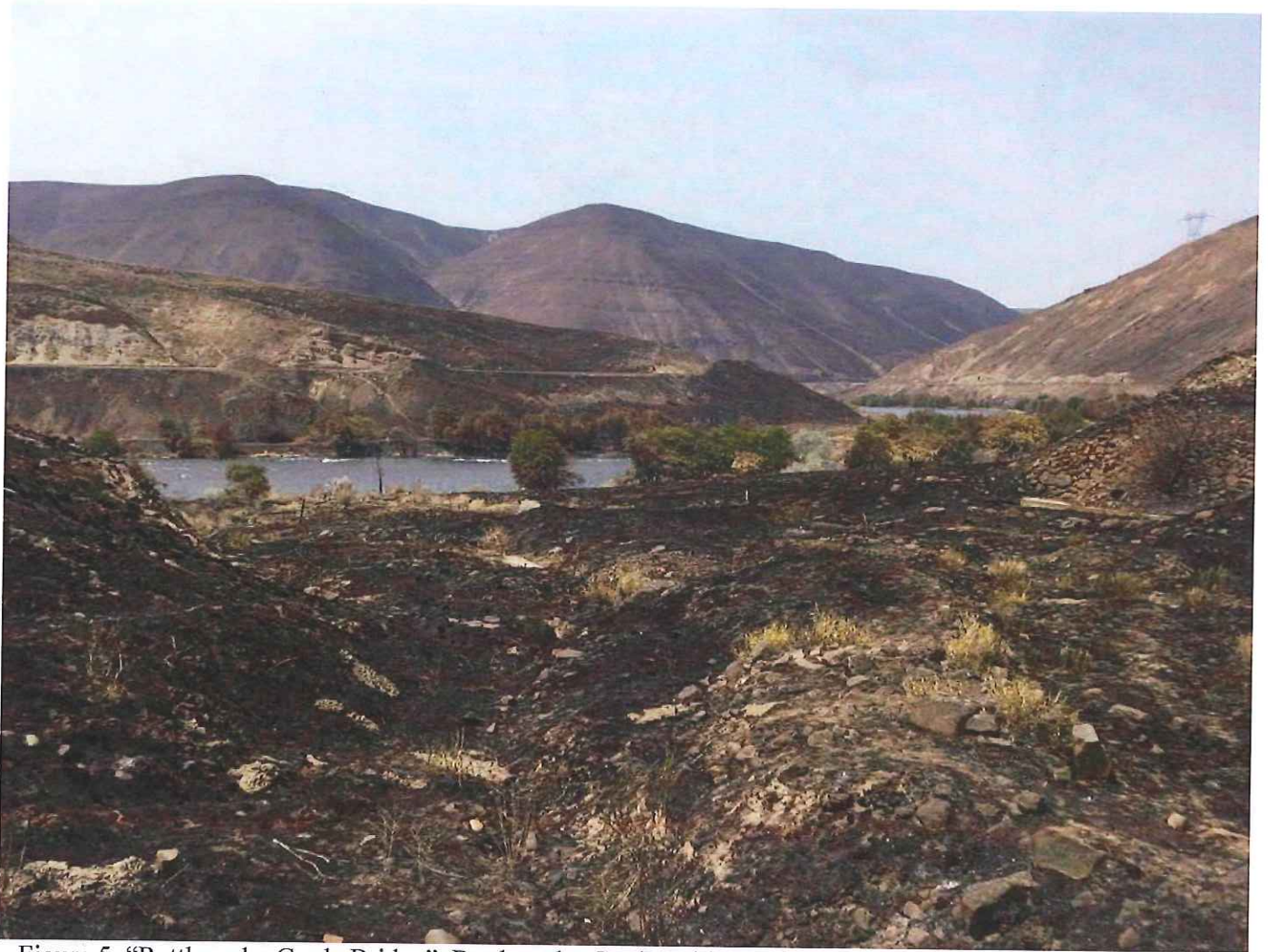
Figure 5. "Rattlesnake Grade Bridge". Rattlesnake Grade Bridge was not previously recorded in the Historic SHPO database, but is presumed to have been part of the historic Harriman railroad alignment. The only portion of the bridge that survived the fire are the earthen bridge approaches and rock rip-rapped abutments. Facing northwest.
