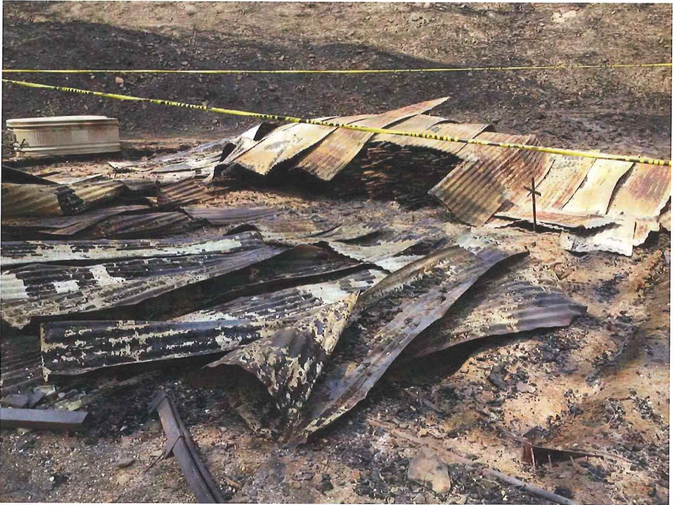
Figure 13. "Harris Ranch Barn/Shed." The Harris Ranch Barn/Shed was completely destroyed in the fire. Facing east.
