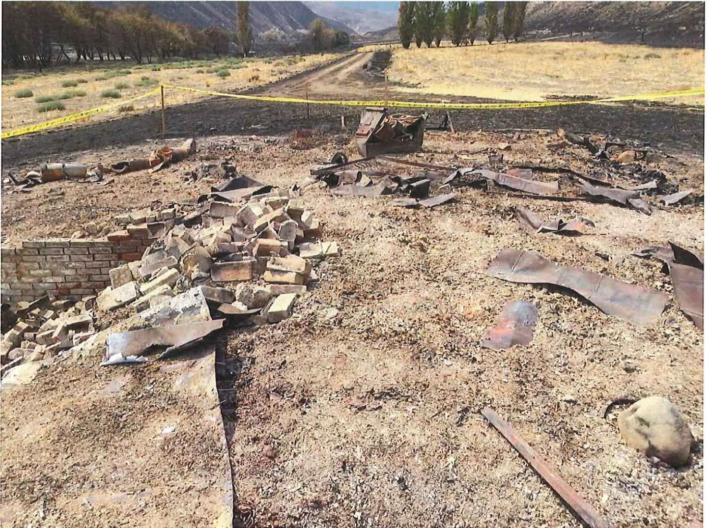
Figure 18. "River Mile 12: Deschutes River Harris Ranch House". Remains of the Harris Ranch House. Facing north.
