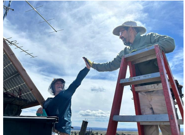
High fives after completing the final install of a Motus tower.
