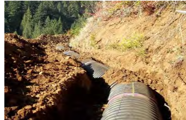
New pipe project
