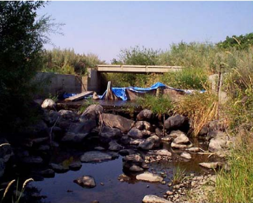
BEFORE: Irrigation dam blocks fish passage
