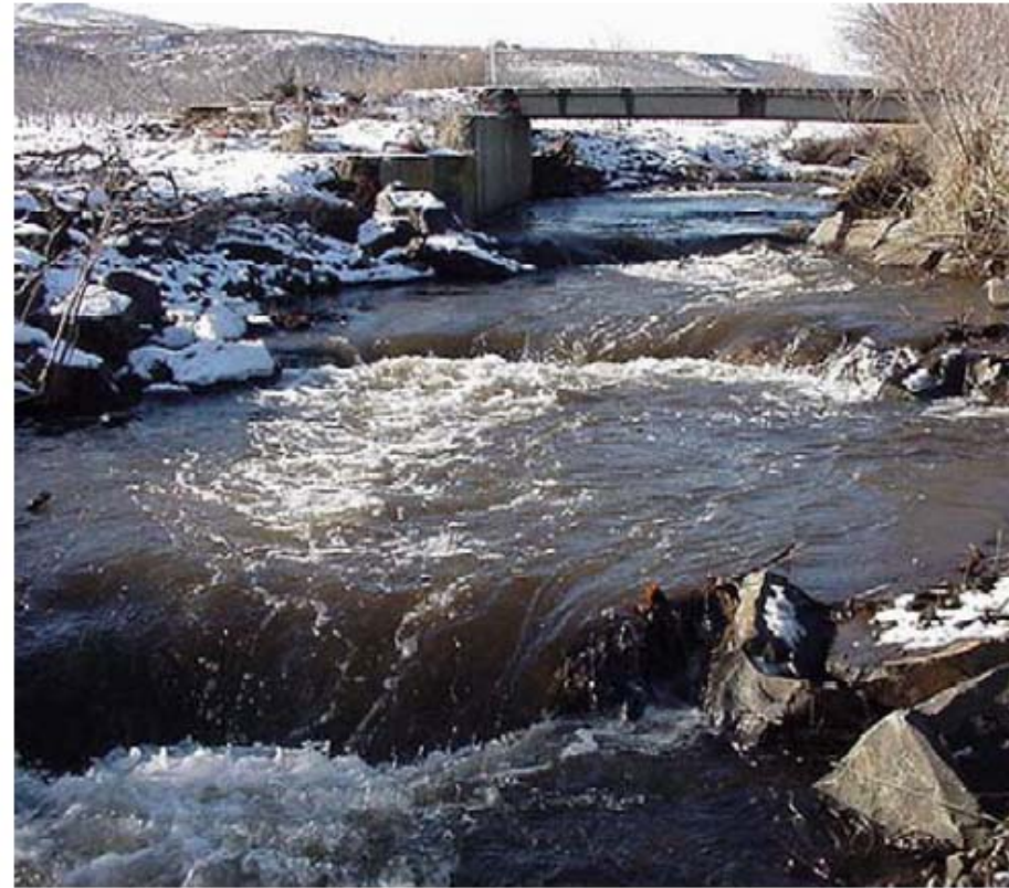
AFTER: Rock weirs allow full fish passage
