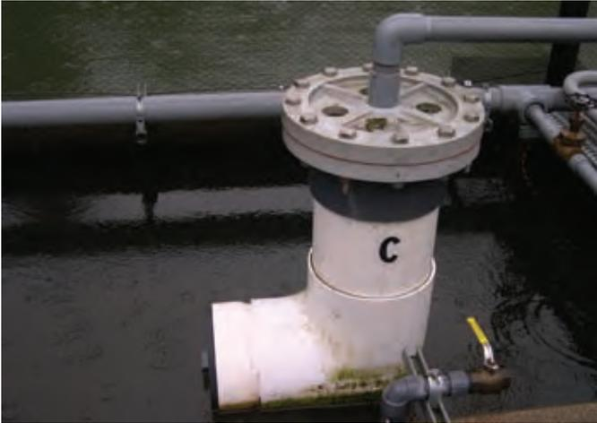
Fig. 4. Air-lift system to recirculate water in stream channels. Compressed air injected through smaller grey pipe lifts water up larger white pipe.
