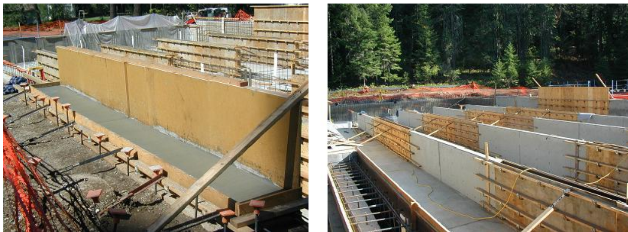
Figure 10. Construction of new raceways at Butte Falls Hatchery.
