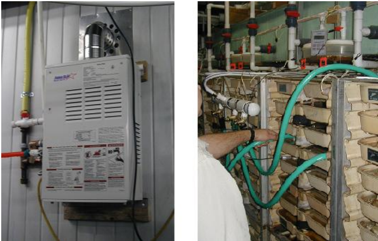
Figure 9. Triploid egg production at Roaring River Hatchery. Left – Propane on-demand water heater used to raise water temperature for shocking eggs. Right – Heated water being applied to eggs in incubation trays.
