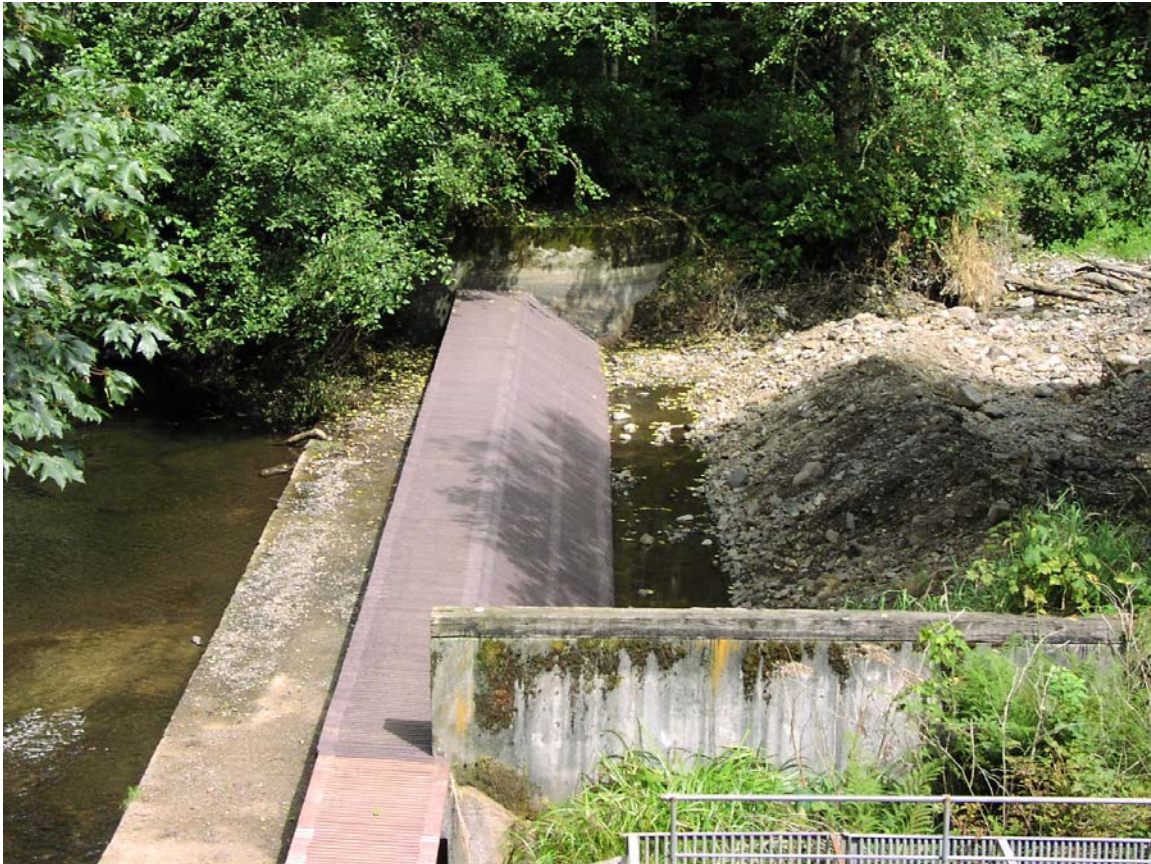
New fish barrier installed at Big Creek Hatchery intake.
