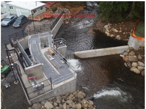
Sandy Hatchery fish ladder and intake
