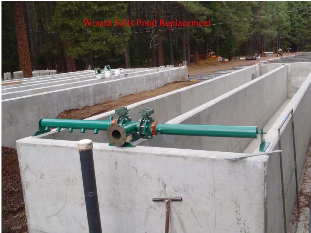
New raceways at Wizard Falls Hatchery
