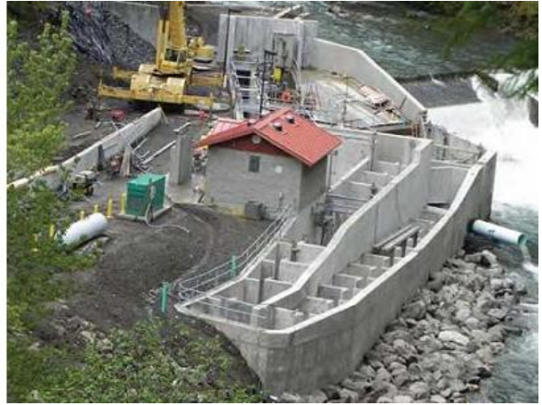
Rock Creek Hatchery fish ladder and intake
