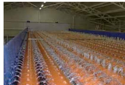
Figure 13. Trickle filter
