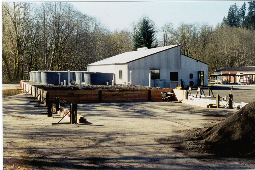
Figure 1. Construction of Abernathy FTC temporary sturgeon facility
