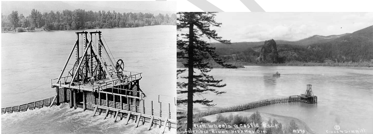
Figure 13a. Left, typical fish wheel used to harvest salmon in the Columbia River Gorge (source: Oregon Historical Society 2018); right, Kelly Fish Wheel, built in 1890, near McCord Creek, Oregon (source: Donaldson and Cramer 1971).
