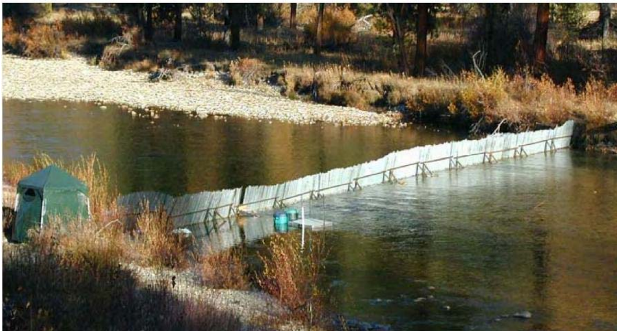
Figure 12c. Example of a fixed picket weir (source: Bureau of Reclamation 2012).
