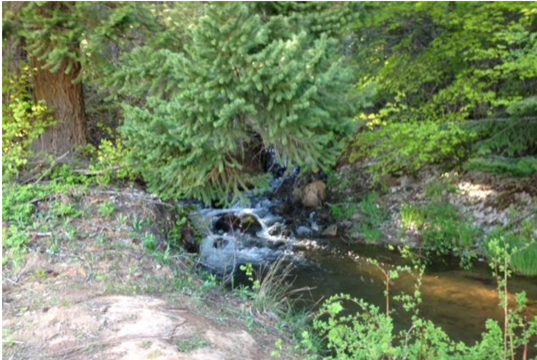
Additional Photo #1. The lower spillway channel of Kingsley Reservoir.
