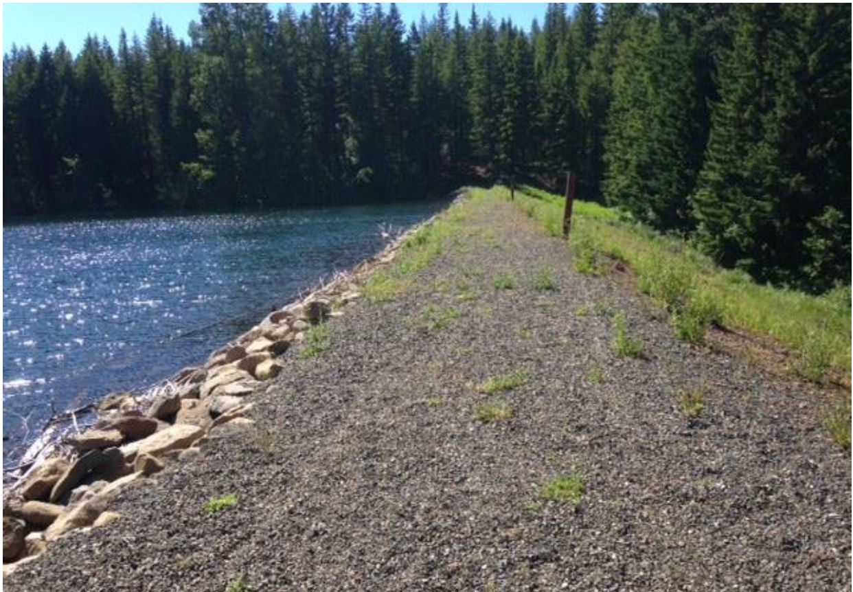
Figure 3. Earthen dam of Kingsley Reservoir.
