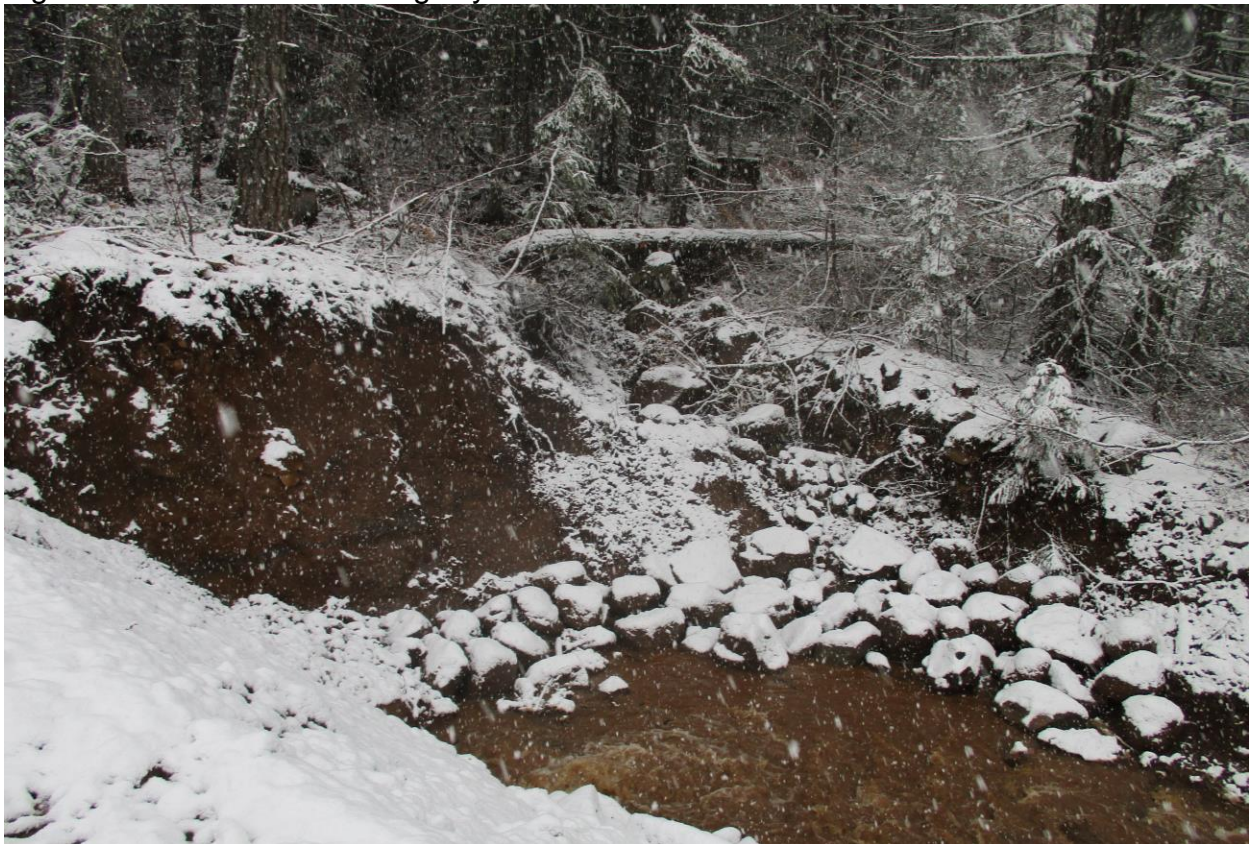
Figure 4. Kingsley Reservoir release pipe and spillway channel.
