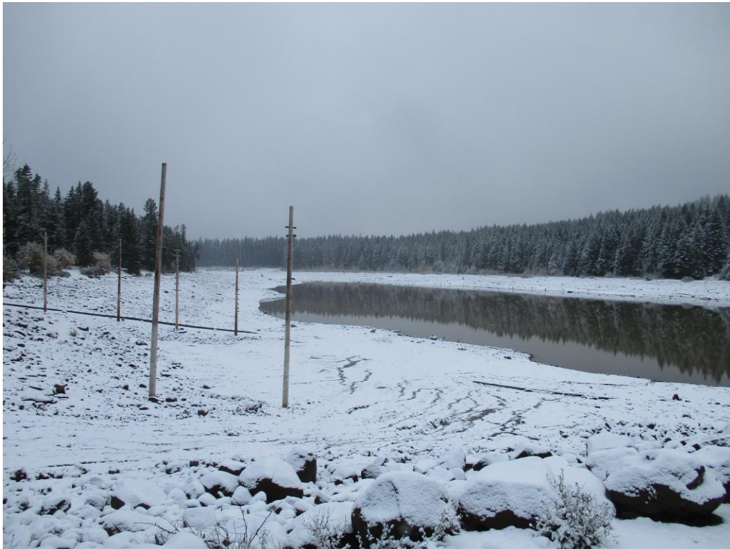
Additional Photo #2. Kingsley Reservoir drawn down for pipe repairs.
