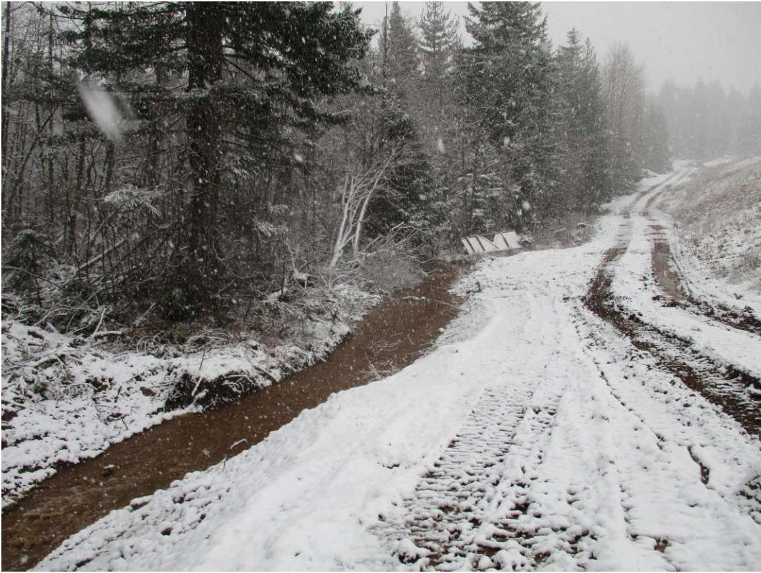
Additional Photo #3. Discharge channel below Kingsley Dam.
