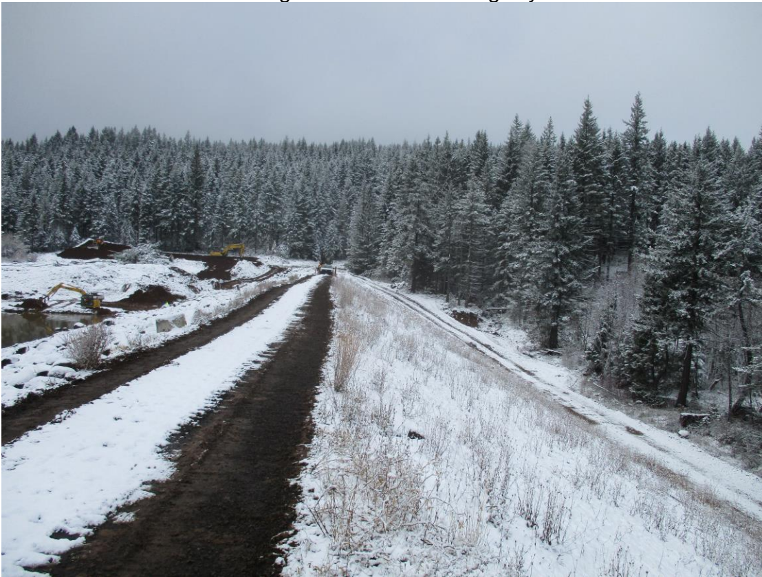
Additional Photo # 4. Backside of earthen dam, Kingsley Reservoir.
