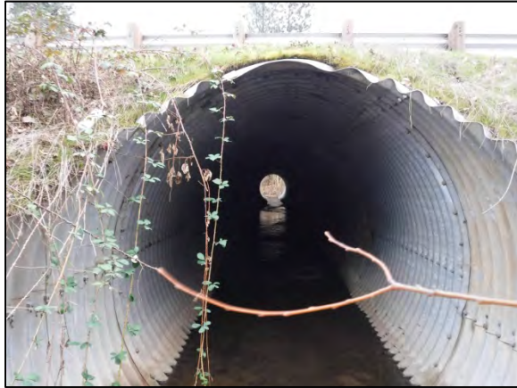
Blackwell Creek Culvert pre-treatment (left), post-treatment (right)
