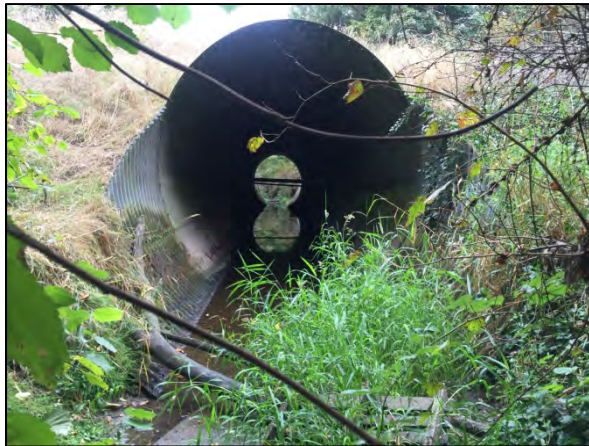
Oakpoint Creek Culvert pre-treatment (left), post-treatment (right)
