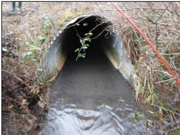
Wilson Creek Culvert pre-treatment (left), post-treatment (right)
