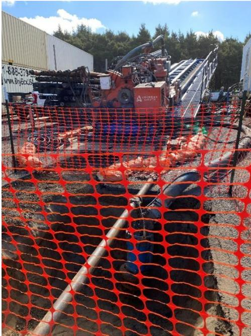
One of two drill rigs set up at Driftwood with drill fluid pump pit. Photo Credit Delia Kelly ODFW, taken with permission from OSU June 9, 2021.
