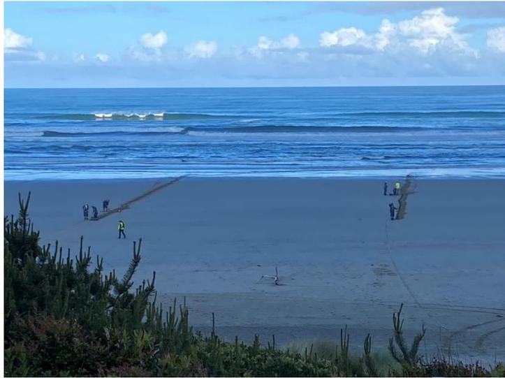
*Wireline installation at Driftwood beach. Cables will be installed beneath the beach between these two wirelines. Photos credit Delia Kelly ODFW taken with permission from OSU June 9, 2021.*
