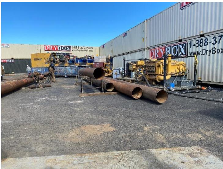
Drill fluid processing equipment and bore hole casings promote bore hole stability and avoid inadvertent release of drill fluid as the drill bores through unconsolidated sediment. Photo credit Delia Kelly ODFW taken with permission from OSU June 9, 2021.
