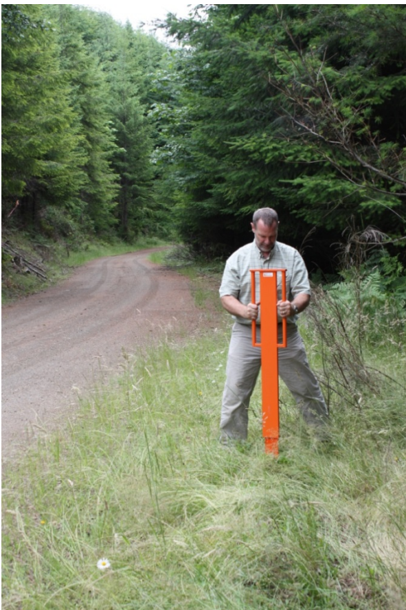
Photo #4. Installation of road markers in 2011, OHA volunteer
